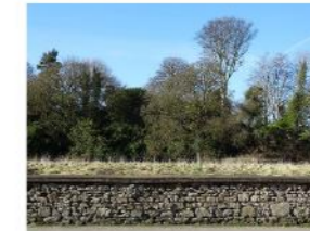
E + F: Fenced off woodland (E) and coursed stone wall against Academy Street (F).
