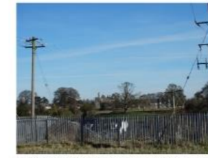
A: Detail of palisade fencing around substation
