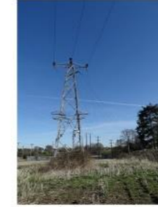
B: Detail of woodland edge adjacent to substation
