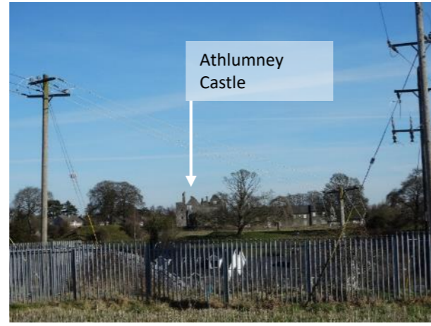
9A. NE over the substation towards Athlumney Castle
