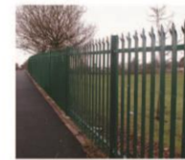
Temporary palisade security fence
