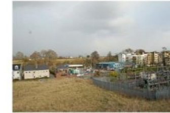
A/U: Palisade fencing around substation (A). Rendered wall against Academy Street (U).
