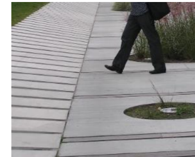
Brushed concrete footpath
