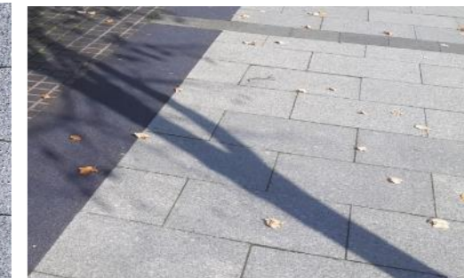
Concrete flags – granite effect
