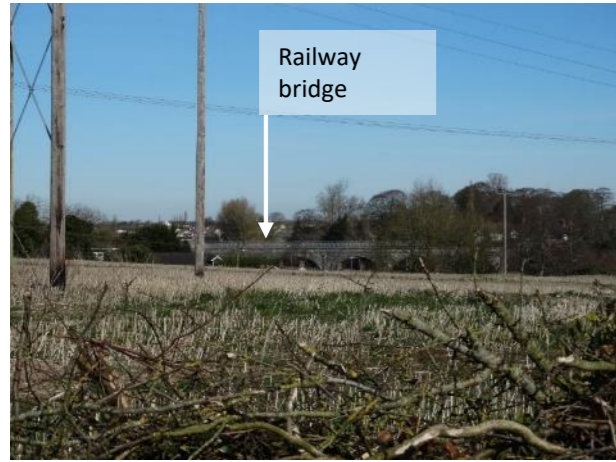
8. View towards railway bridge
