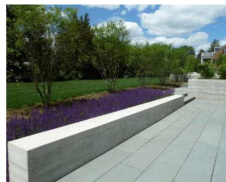
Concrete seat wall
